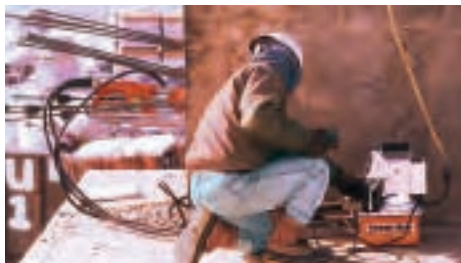
The PE60 used for pre-stressing.
