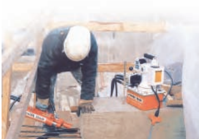
The PE60 used for pre-stressing.
